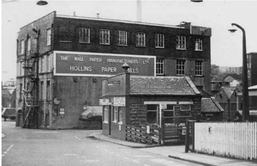
Photograph of historic former factory building on the site
