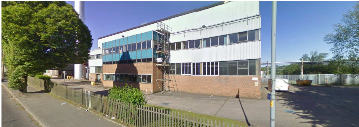
View of the Site from Lower Eccleshill Road Prior to Demolition
