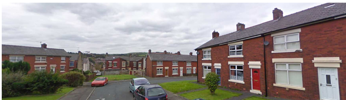
View of existing red brick semi detached and terraced properties just behind the above properties
